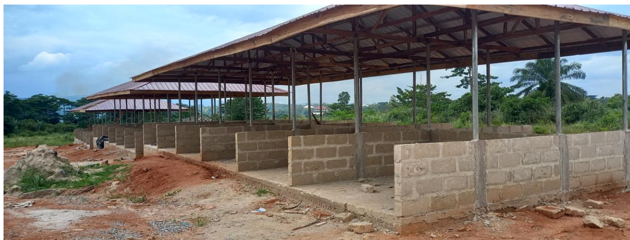
Construction of Lockable Market Stores At Agona
